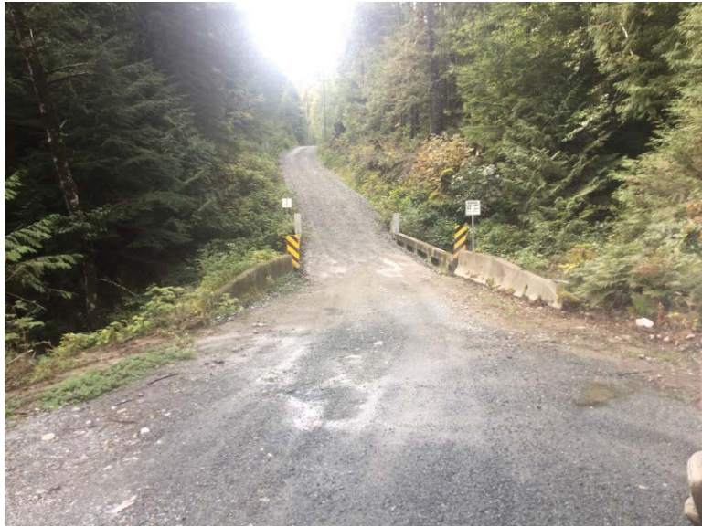
Approach from Right Bank when facing downstream
