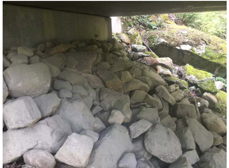
Left Bank Abutment when facing downstream
