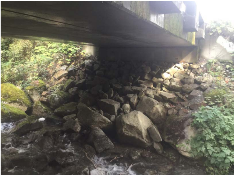
Right Bank Abutment when facing downstream
